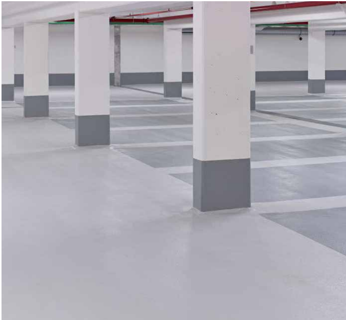
Parking podziemny Platz d’Agen, Dinslaken, DE Systemy StoCretec: StoConcrete Repair Prime TS 100, StoConcrete Protect V, StoFloor Traffic DV 100 Fot.: Guido Erbring
